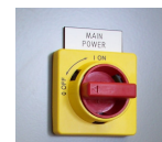
Figure 3-2 Main Disconnect
