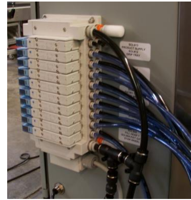
Figure 6-3 Air Solenoids
