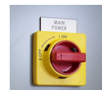
Figure 3-2 Main Disconnect
