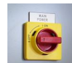
Figure 3-2 Main Disconnect
